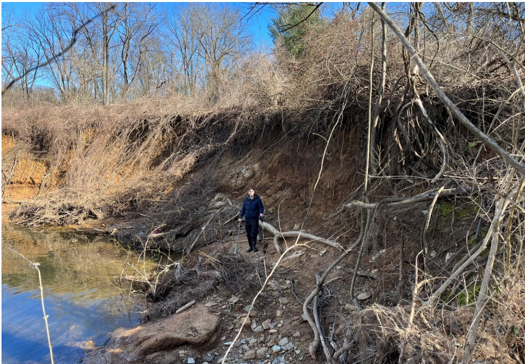
Pictured: Severe streambank erosion along project reach, February 7, 2024.
