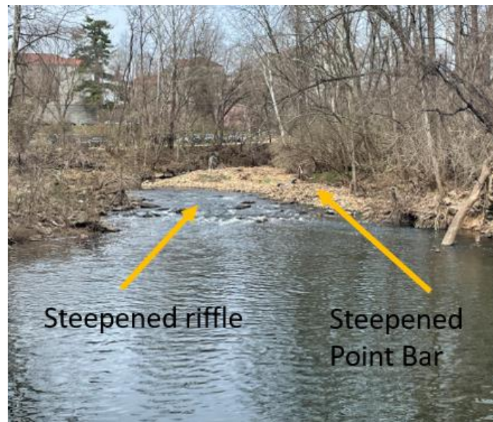
Figure 9: Observations of steepened riffle and point bar faces are diagnostic of active vertical adjustment, suggesting that the erosion problems within the reach are likely to worsen over time as incision leads to increases in bank height and mass failure. Downcutting will also increase the production of coarse bed load which will increase downstream point bar formation.
