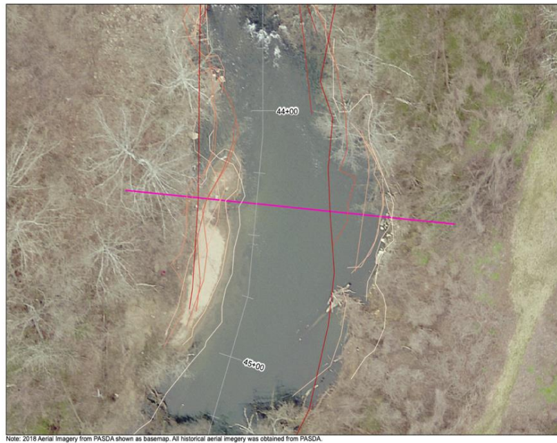
Figure 3: Aerial photograph analysis showing bank retreat along an outer meander bend within the study reach. The dark lines indicate the location of the stream banks in 1996, while the lightest lines indicate the position of the banks in 2020.
