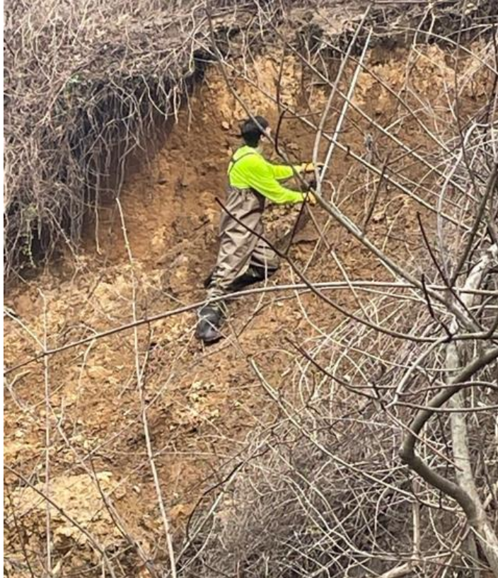
Figure 1: Photograph showing extreme bank heights within the project area. These conditions are unusual compared to conditions found elsewhere along the Wissahickon and extreme when compared with regional data, creating an optimal opportunity for a concentrated and immediate water quality benefit. This bank has retreated by an additional several feet during relatively small storm events this spring. Erosion is occurring into an adjacent hillside with no riparian zone, so bank height will further increase as the erosion proceeds.
